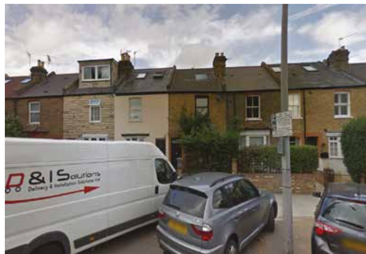
Resi - West of Site - Adhoc Alterations
