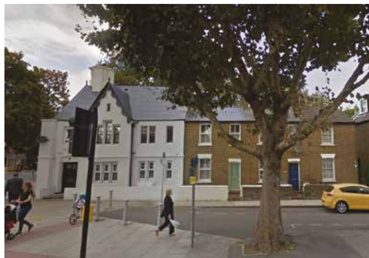
Resi - 2 Storey - East of Site
