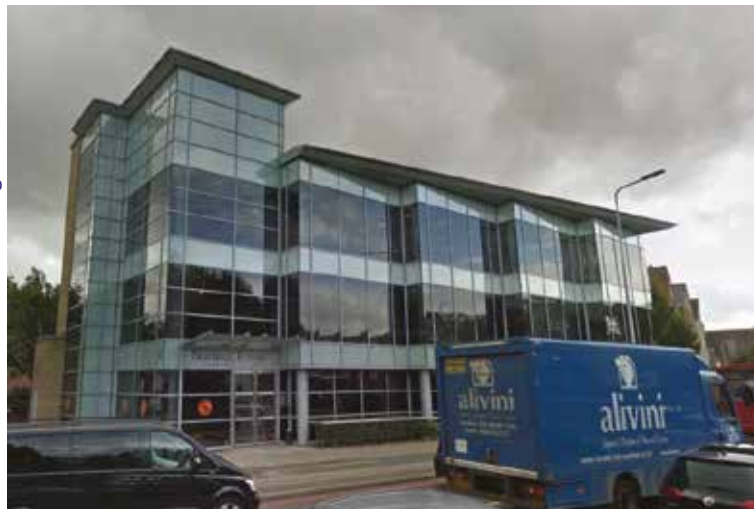
Commercial - Modern Buildings
