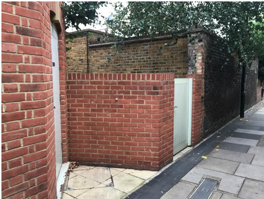
Appendix 2.4. Photograph showing the recent development at the northern extreme of Blue Anchor Alley (which provides precedent for the proposals)
