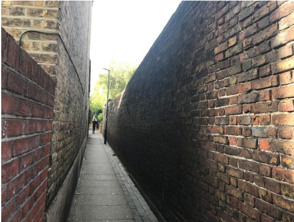
Appendix 2.5. Photograph showing the view along Blue Anchor Alley (the Site is located on the right)
