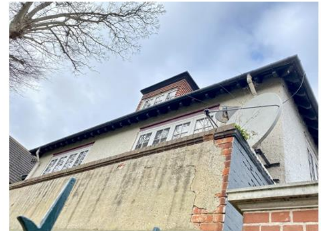
Picture 6: Looking up at the eaves along B1's southern elevation.
