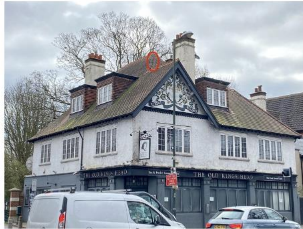
Picture 1: B1's northern and eastern elevations.
