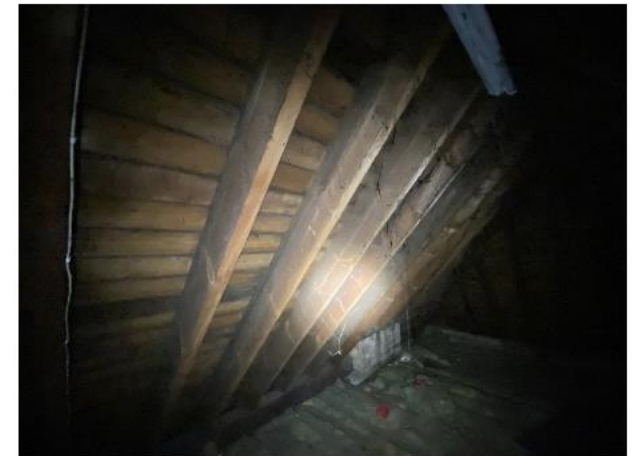
Pictures 15 & 16: Inside B1's loft space, facing north-east and south-east, respectively.
