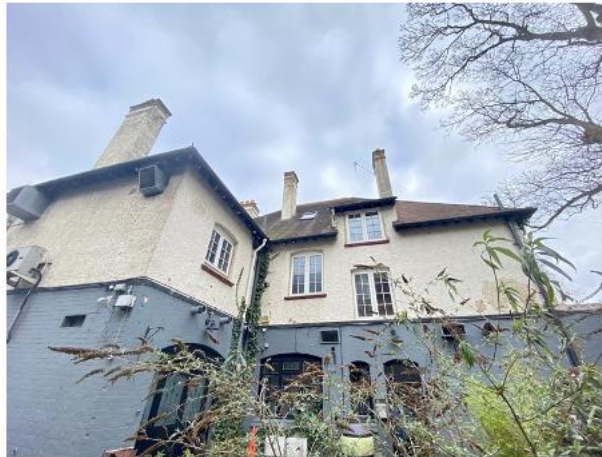
Picture 7: B1's western elevation.
