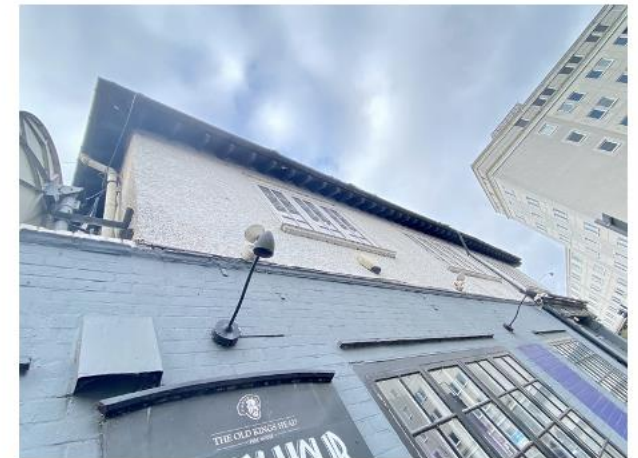
Picture 4: Looking up at the eaves along B1's eastern elevation.
