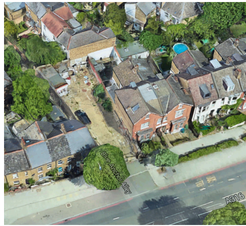
View from the South
