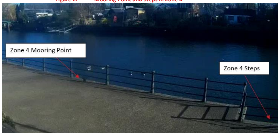
Figure 2. Mooring Point and Steps in Zone 4
