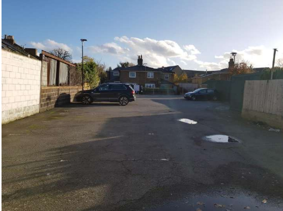
Photo 6: Photo of drain by entrance of car park.
