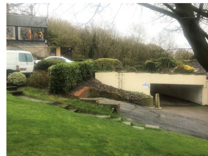
Fig 6 - View of car-park entrance
