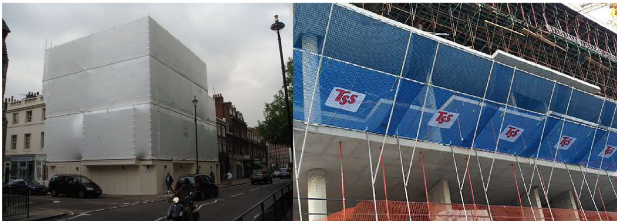
Figures 11 & 12: Full Building Scaffolding and Safety Fans
