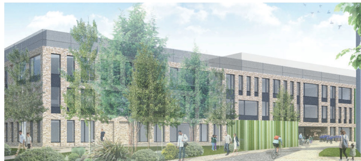
Current proposed facade with brickwork, variation in window height and width but with a vertical emphasis
