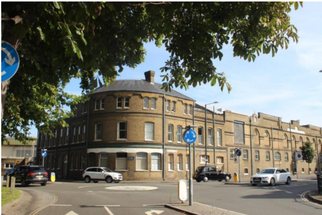
Former Hotel Building
