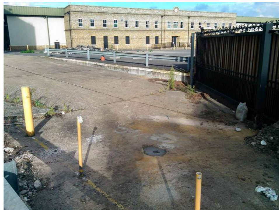
Photograph 10. Typical completed borehole
