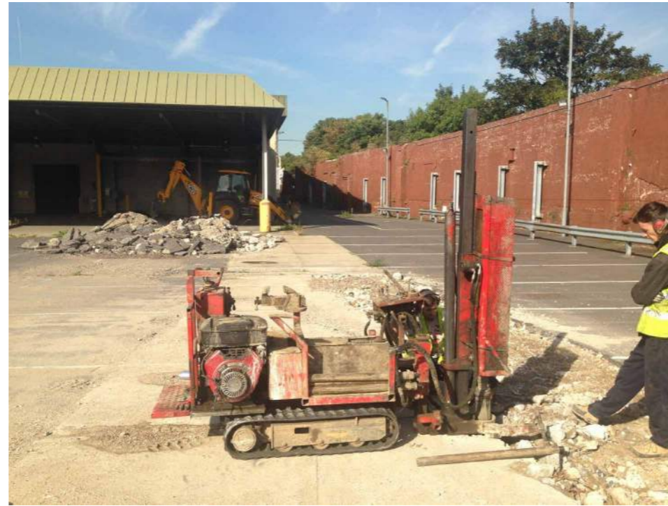
Photograph 7. Ground investigation works in progress
