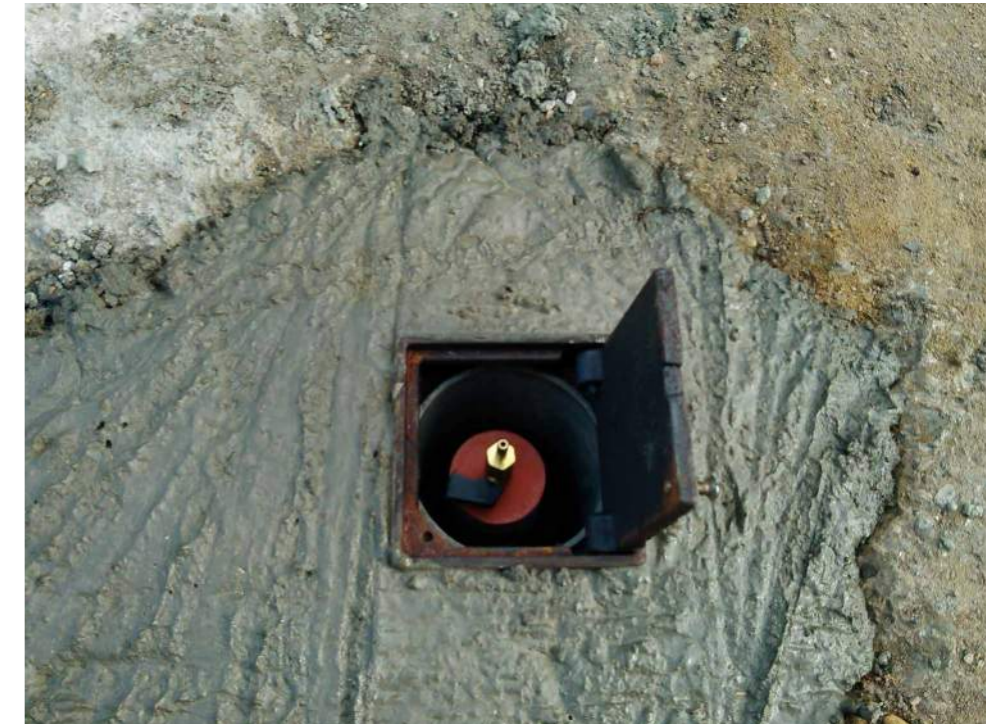
Photograph 8. Typical completed borehole
