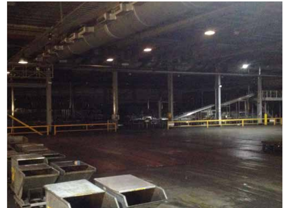
Photograph 3. Interior of packaging warehouse
