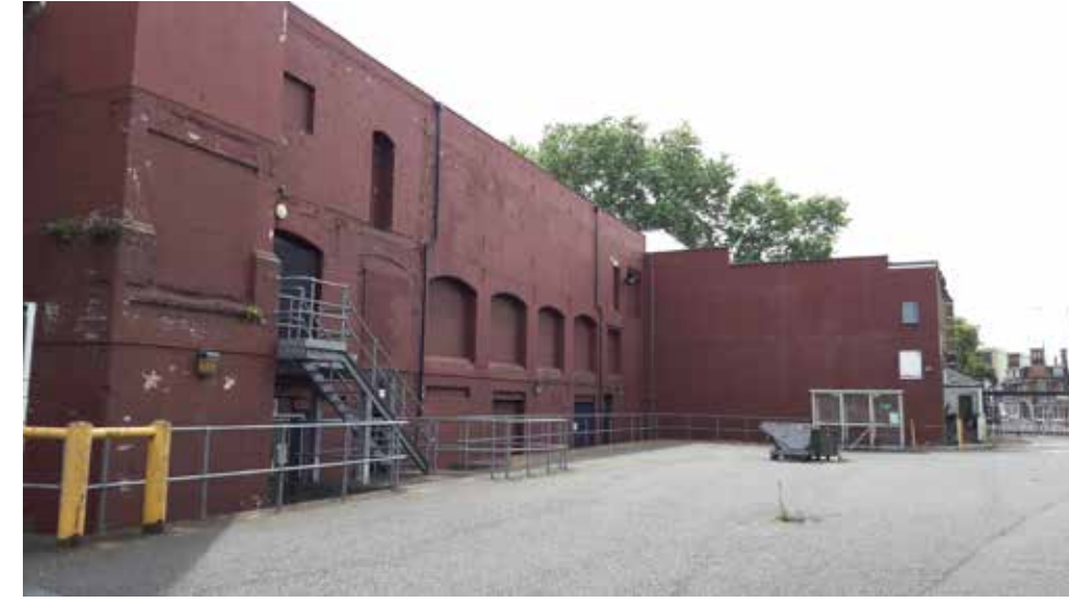
Photo 4 Former Hotel and Former Bottling Hall
