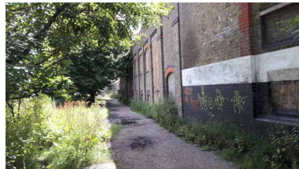
Photo 3 The Site perimeter wall from the tow path
