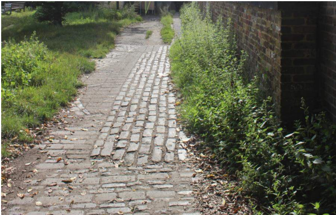
Plate 31: Granite paving setts (2017)
