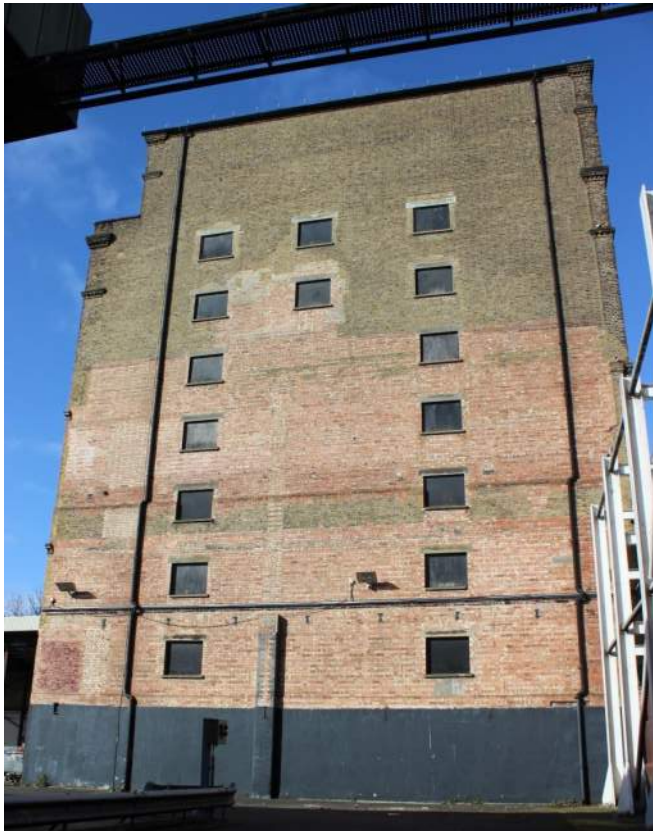
Plate 13: East facing elevation of Maltings
