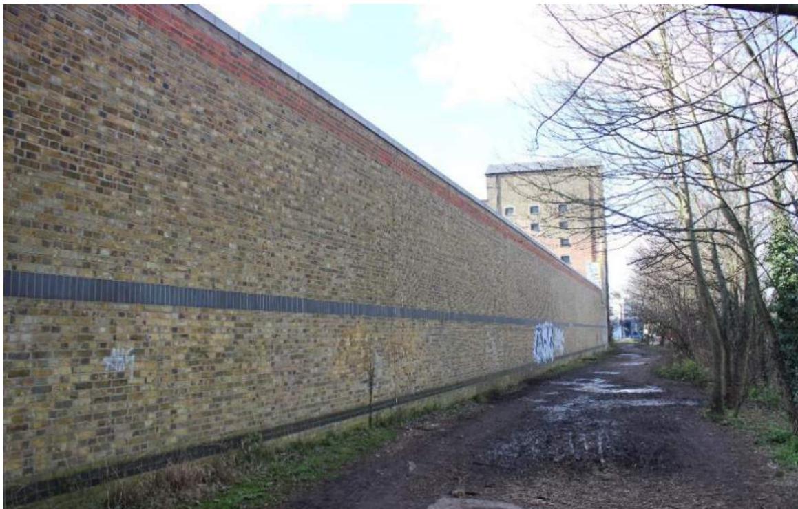
Plate 16: Section 1 - Late twentieth century wall (2017)
