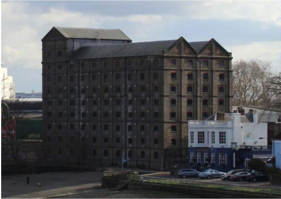
Plate 12: West facing elevation, as seen from Chiswick Bridge (2017)
