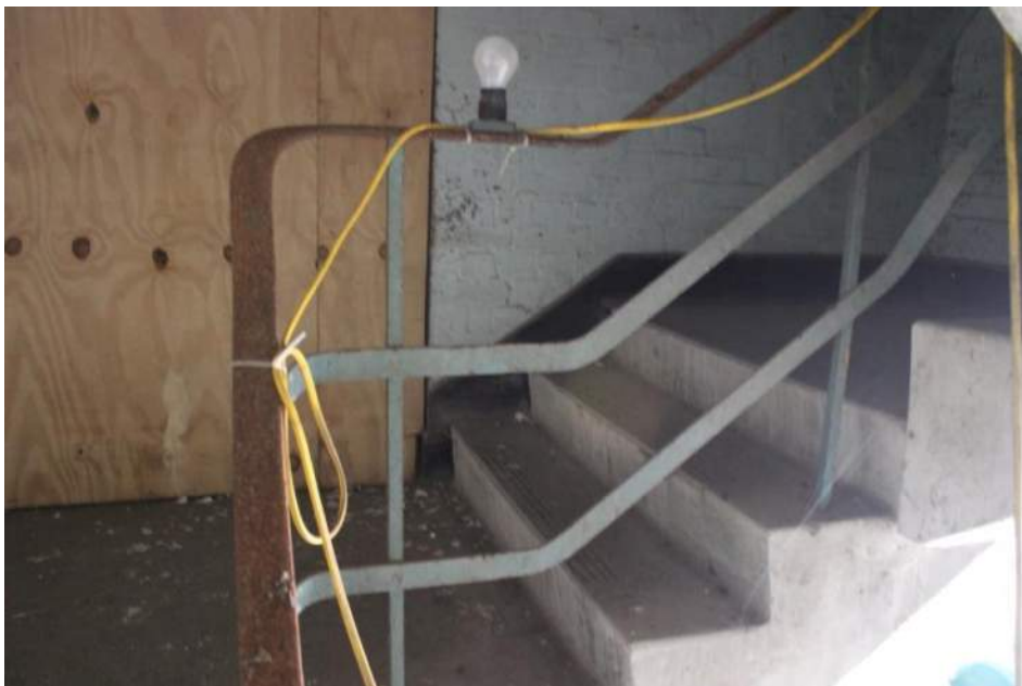
Plate 15: Staircase to interior of Maltings building
