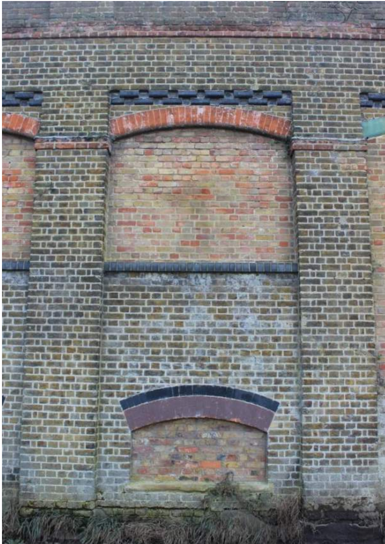
Plate 19: Part of the wall in Section 4 (2017)
