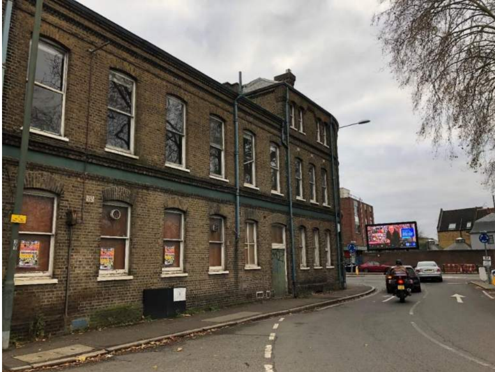
Plate 2: West facing elevation of Former Hotel (2021)
