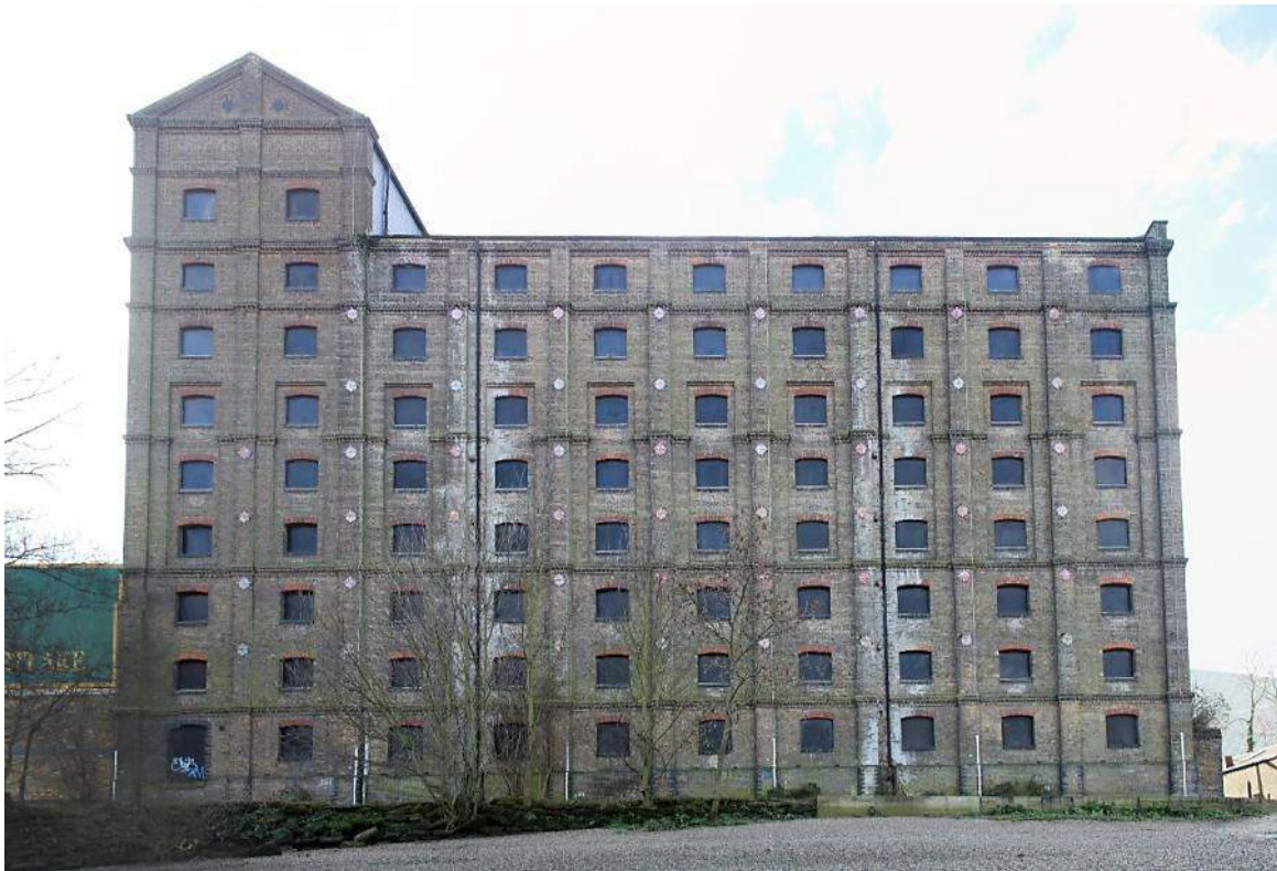
Plate 10: North facing elevation of Maltings (2017).
