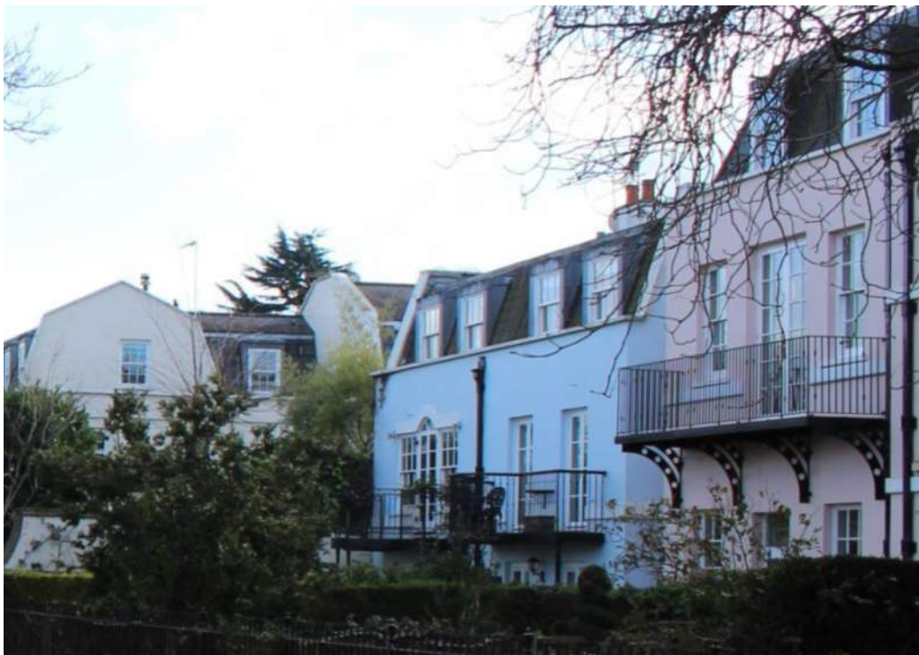
Plate 41: Building of Townscape Merit 6 and 7 Thames Bank and corner of Grade II Listed Riverside House (2017)
