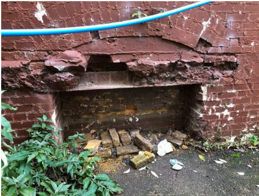
Plate 26: Interior elevation of north boundary wall (2021)
