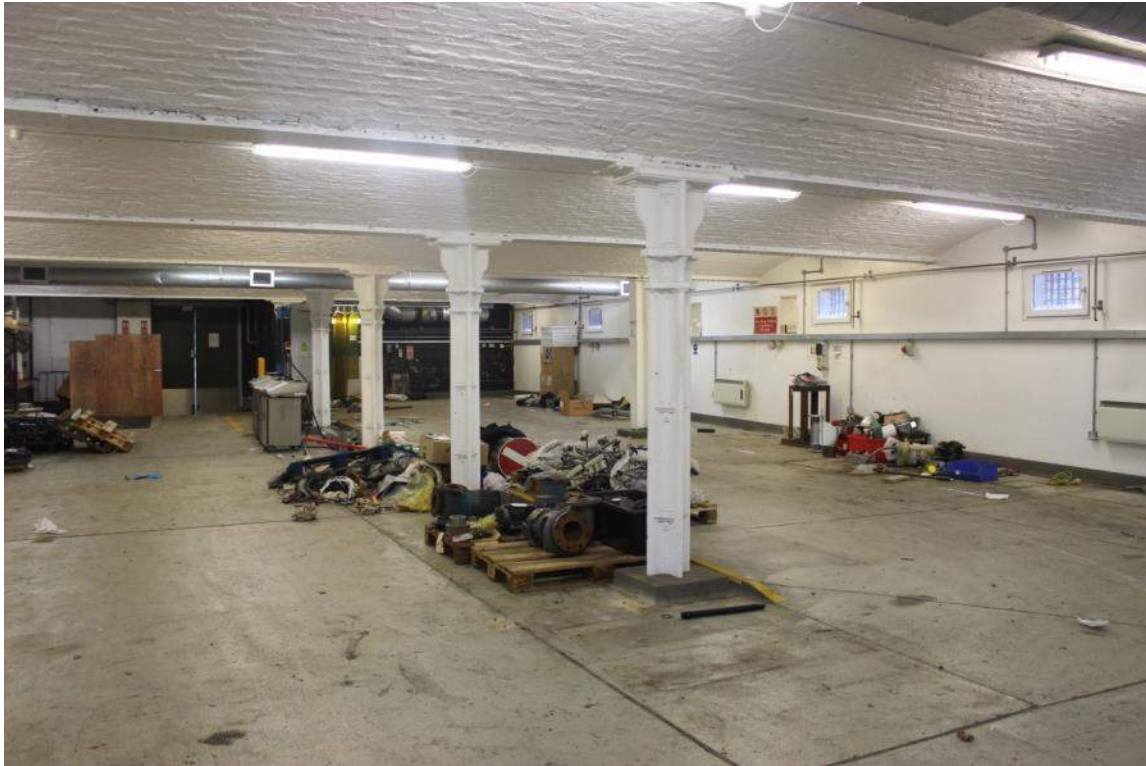
Plate 7 Interior of sub-ground floor of former Bottling building, illustrating brick arches and cast iron columns (2017)
