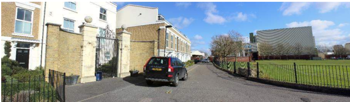
Plate 45: Grade II Listed Building Gates to Cromwell House within their setting (2017)
