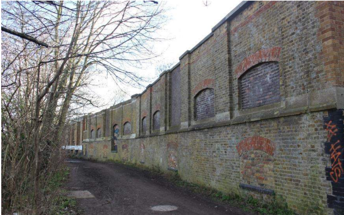
Plate 17: Section 2 - Mid 19th century wall (2017)
