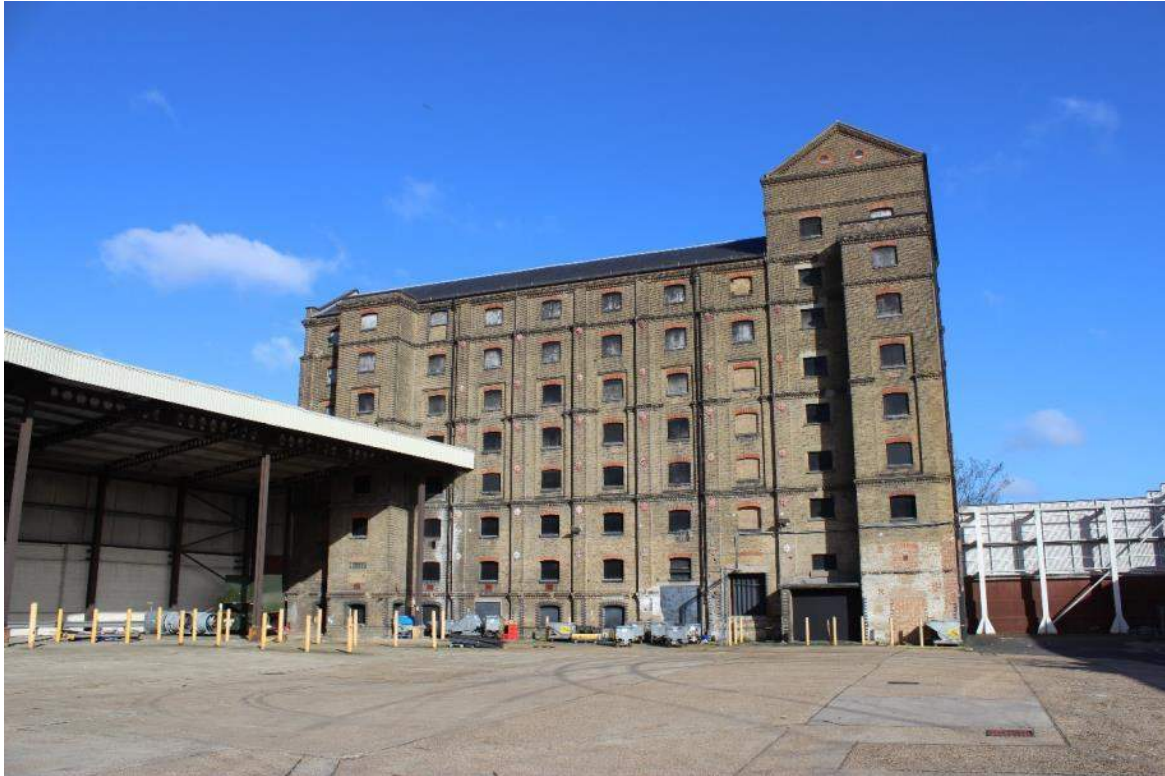
Plate 11: South facing elevation of Maltings (2017)
