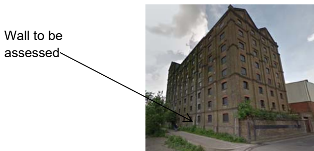
Figure 3: Wall to be assessed
