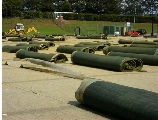
Rolled carpet ready for removal
