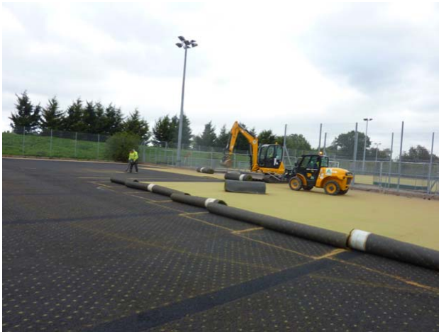
Rolling up carpet – limiting damage during process
