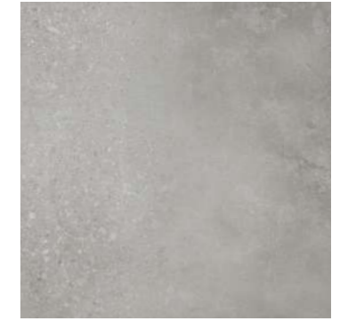
6. Concrete with exposed aggregate
