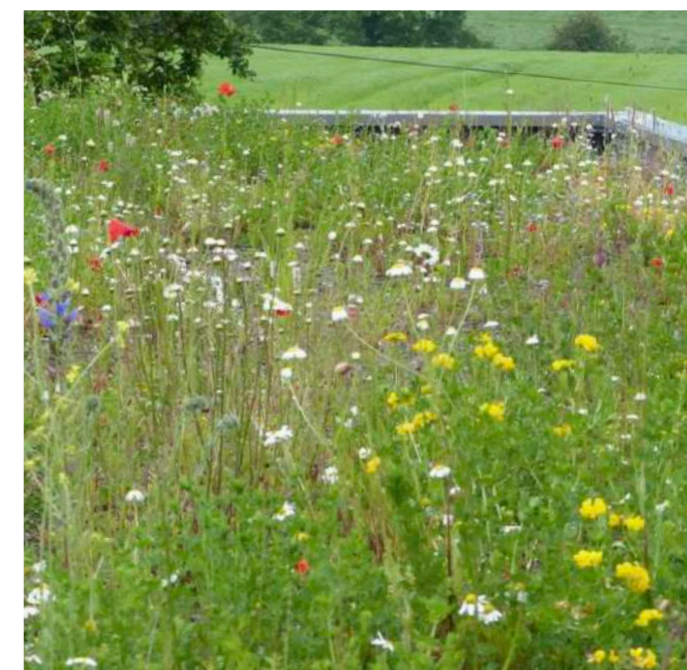
A Wildflower green roof provides biodiversity, drainage attenuation & enriches the landscape setting of the CA
