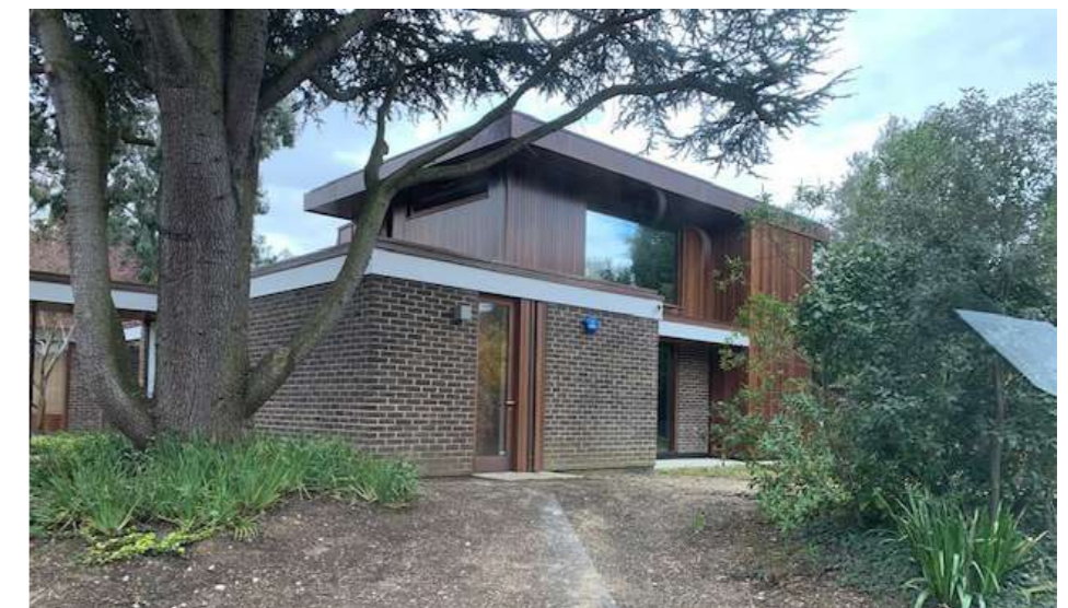
The street hosts a variety of different designs dating from the 1950s, including this locally listed property at 7 Ham Farm Road, recently extended.
