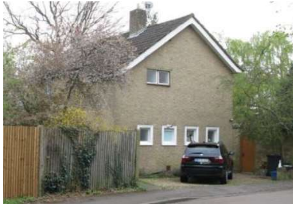
6 Ham Farm Road: Original Dwelling
