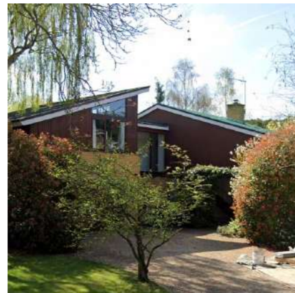
Reference: dark stained timber cladding in local properties of townscape merit, such as 21 Ham Farm Rd
