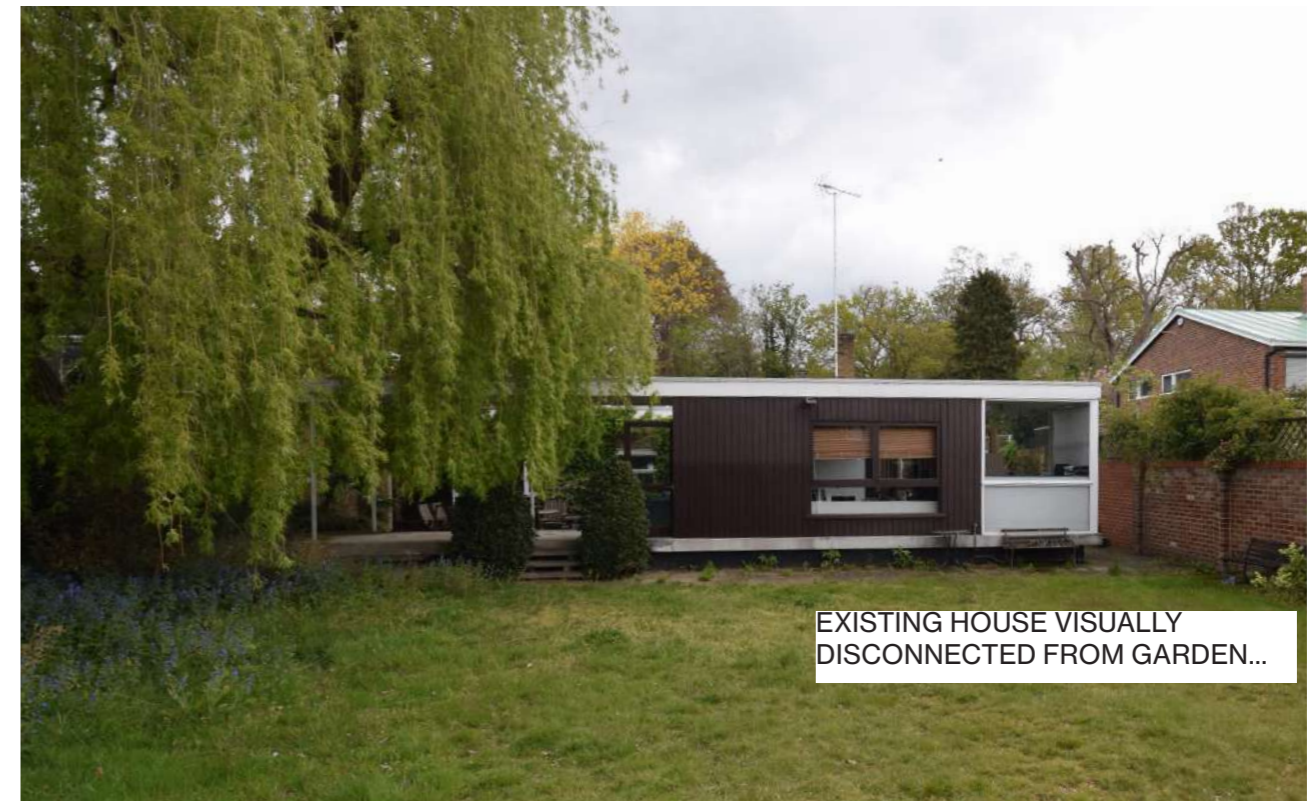
25 Ham Farm Road: Garden Elevation: discordant design between front and rear of dwelling
