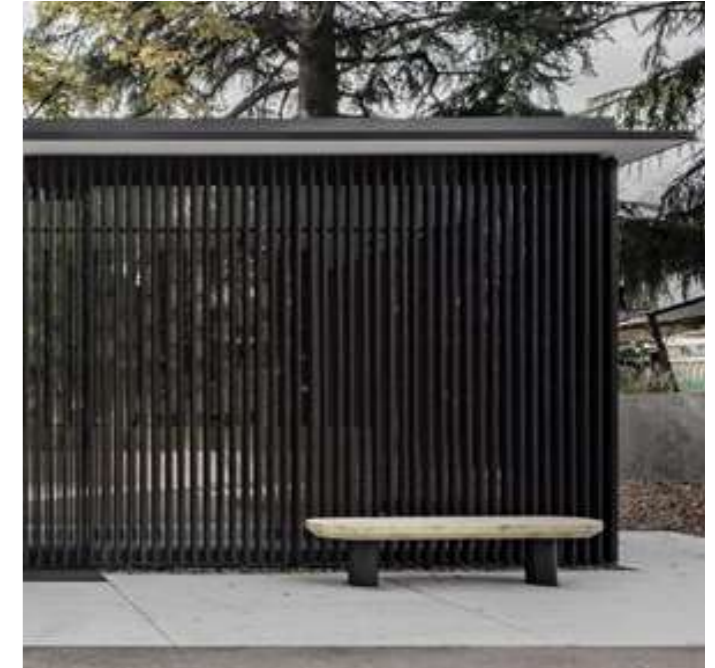
Textural vertical cladding provides character, modulates views for privacy and is sustainable.
