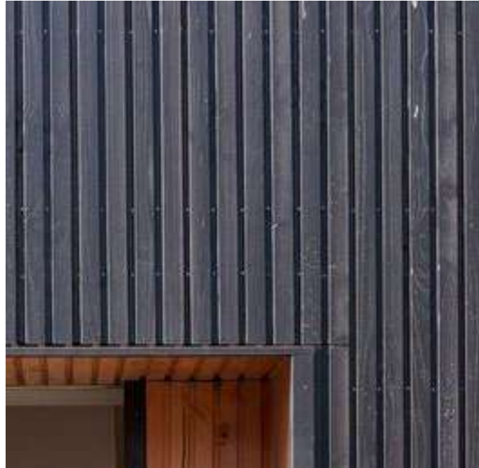
Dark stained timber builds on the tradition of stained timber cladding in the locality, adding character & natural longevity.
