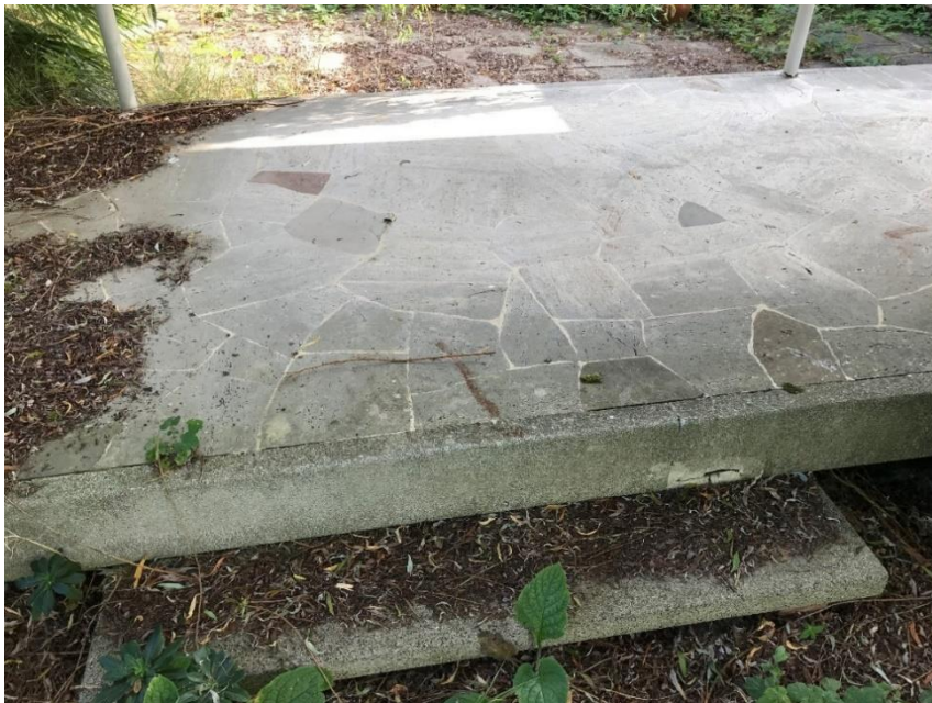
Figure 8: crazy paving to the covered linear terrace formed from broken marble (No. 25)
