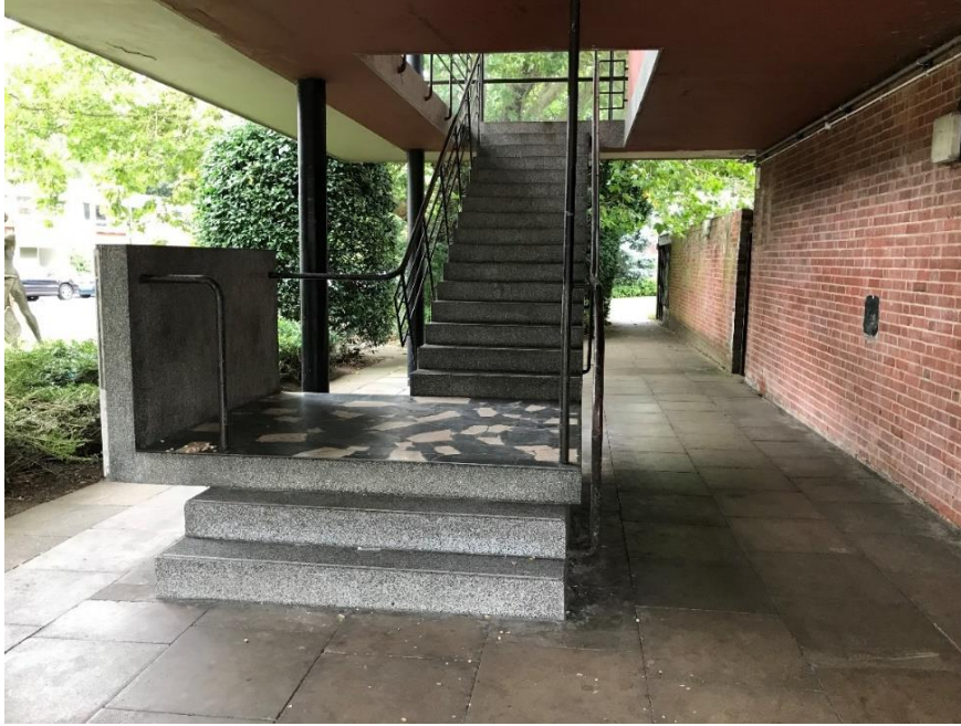
Figure 9: Dryden Court – staircase to flats at the upper level
