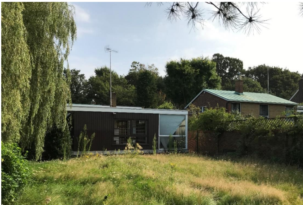
Figure 12: View of No. 25 Ham Farm Road from the south west (rear garden). No. 27, by Bernard Kreeger (1956) is to the right.
