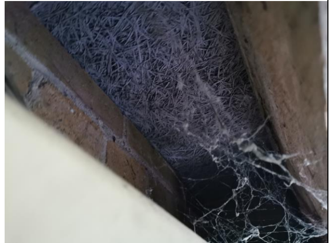
Photo 14: Garage loft void.
