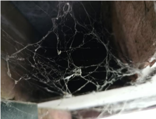
Photo 15: Garage loft void.
