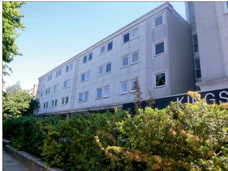
Photograph 1: Showing the front of the building.
