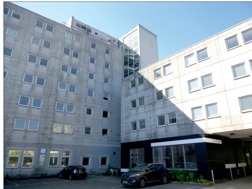
Photograph 2: Showing the rear of the building.
