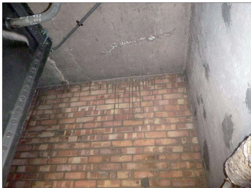
Photograph 3: Showing the well-sealed service unit.
