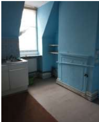
4.7 The Kitchen fireplace has been covered and the boiler condensing waste pipe placed across its front, needs to be removed and the original interior shown if it is still there. This will become the Tea room for the offices.
