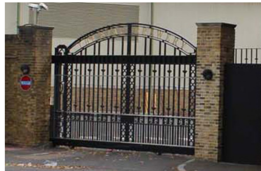
Stag Brewery Gate 1 - from one side of main entrance on Lower Richmond Road (5.0m wide)
