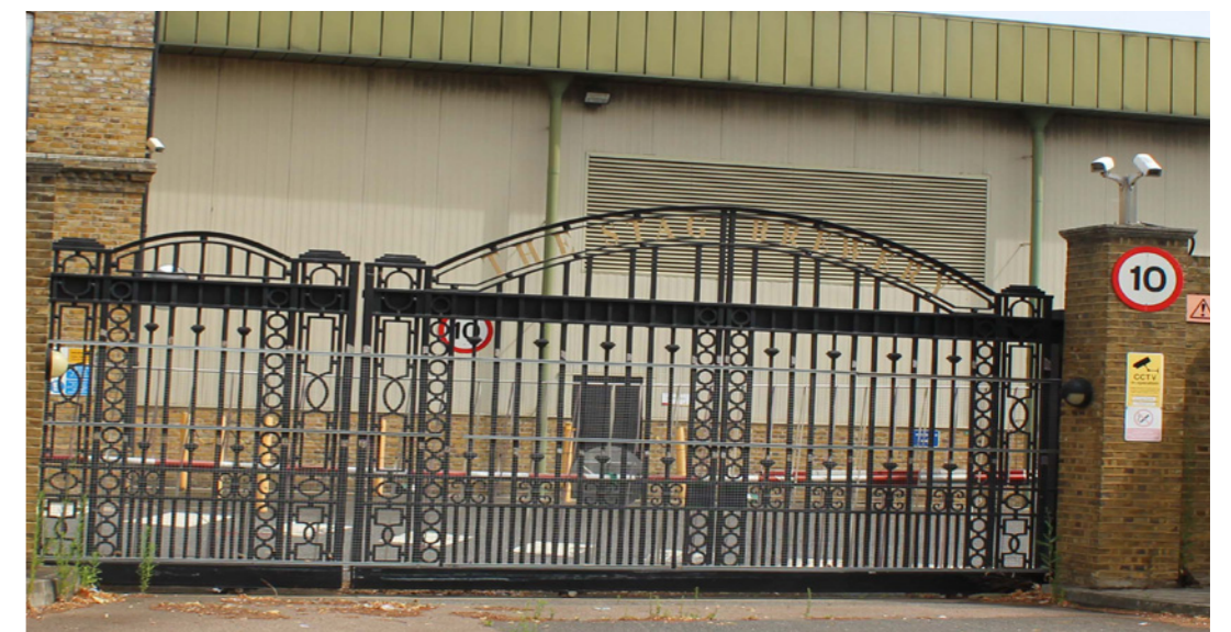
Stag Brewery Gate 2 - main entry gates from Lower Richmond Road (7.0m wide)
