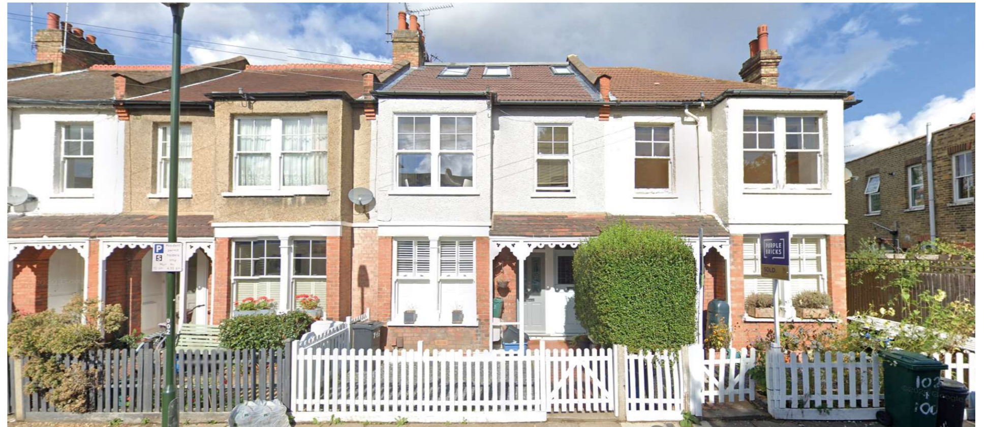
1-7 Godstone Road Houses - North Of The Car Park Site
