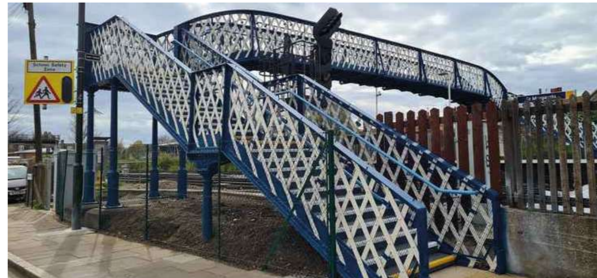
St Margarets Footbridge
