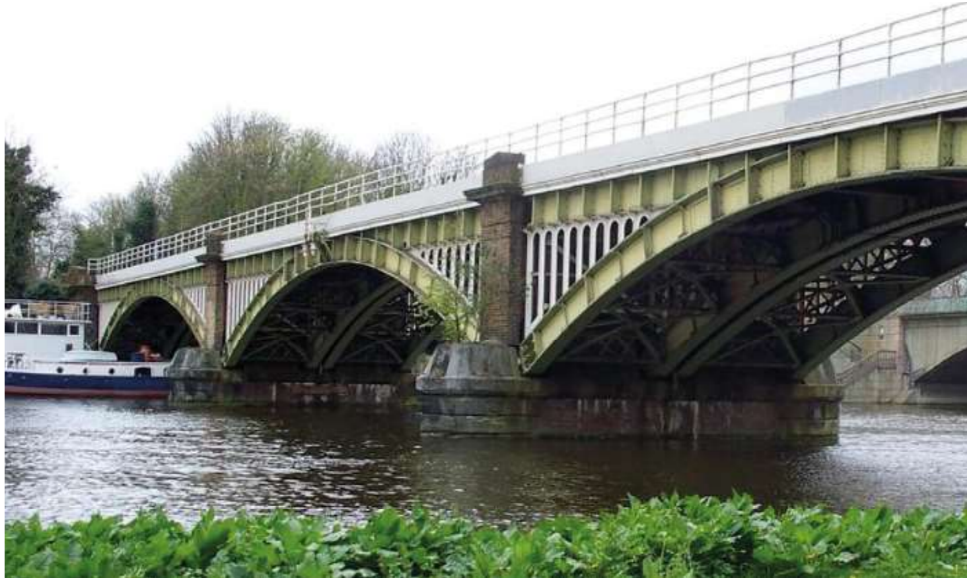
Richmond Railway Bridge
