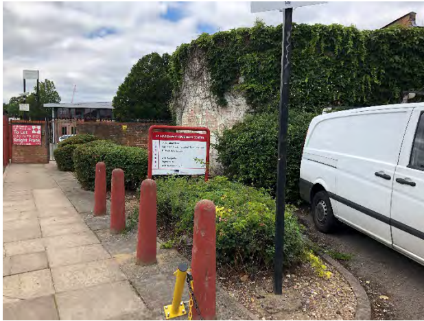
Photograph 3.5 Ivy clad wall on western site boundary
