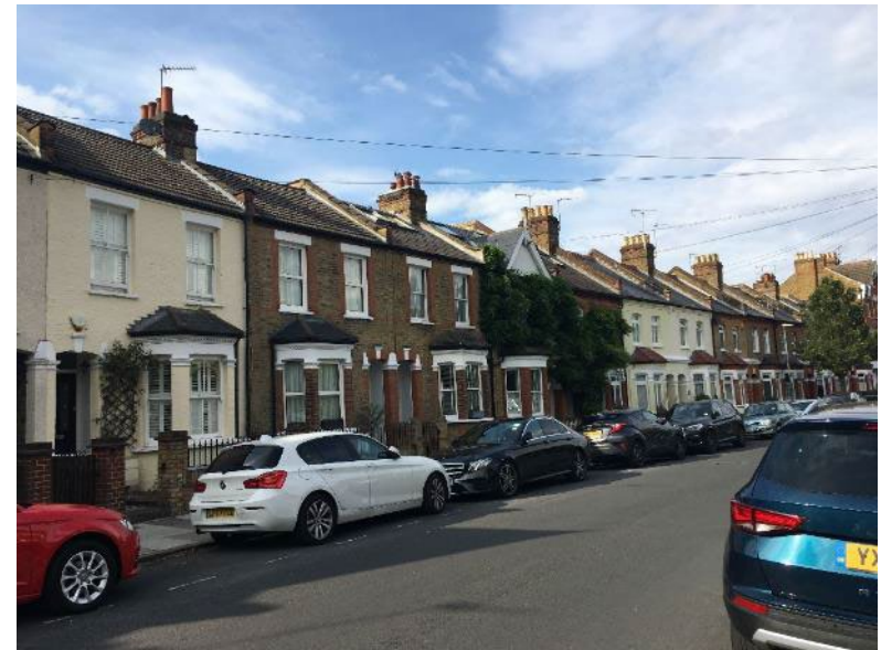
Plate 15: Terraced housing on the north side of Amyand Park Road.
