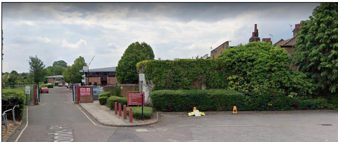
Figure 3 - Gated Access to St Margarets Business Centre
