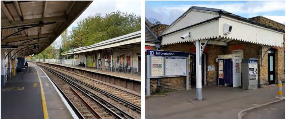
Figure 4-9: Mortlake Station Platforms and Its Southern Entrance
