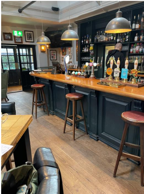
Engineered timber planks in bar area
