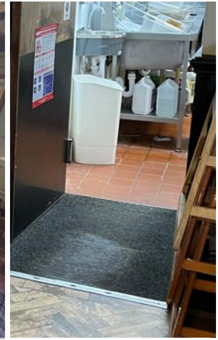
Barrier matting and terracotta tiles in kitchen
