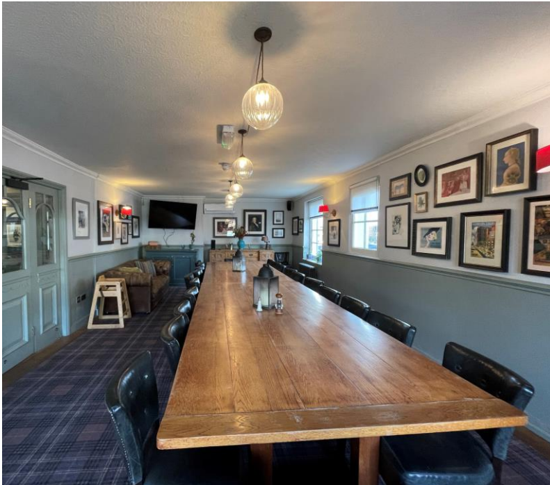
Plain Dado panelling to walls of function room.
