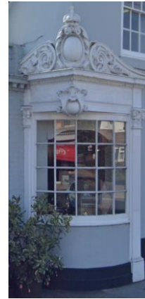
Plaster ornament to corner window
