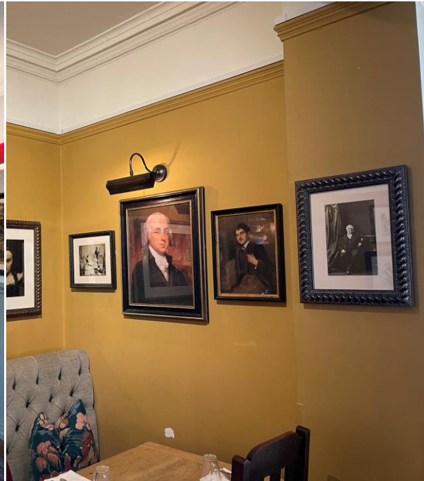
Simple corning and picture rails, seen in the bar "flex" area.
