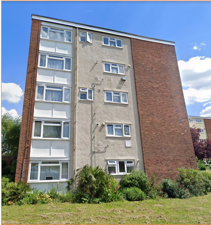
Figure 12: Existing Edwards House.
