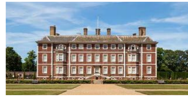
4 Ham House was completed in 1610. It is Grade I listed with a mix of early Jacobean English Renaissance and classical style architecture.
