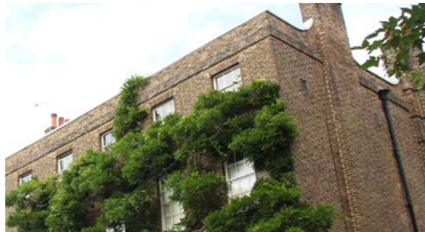
Langham House (Rear) - Grade II Listed Building
