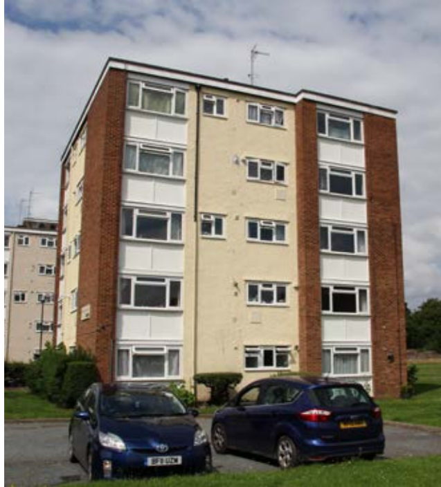
5 storey block with parking court in foreground
