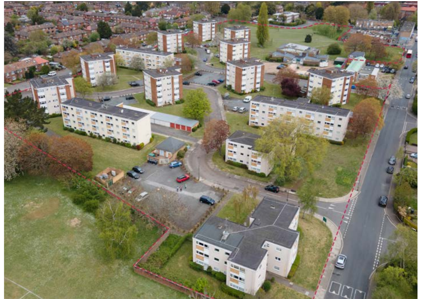
Aerial view looking east from the south west corner of the site
