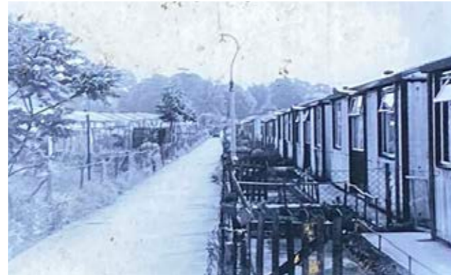
View down Woodville Road towards Beaufort House.
