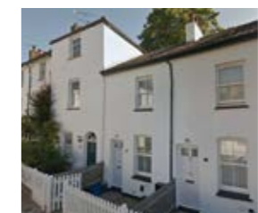
Ham Street Stepping roof line
