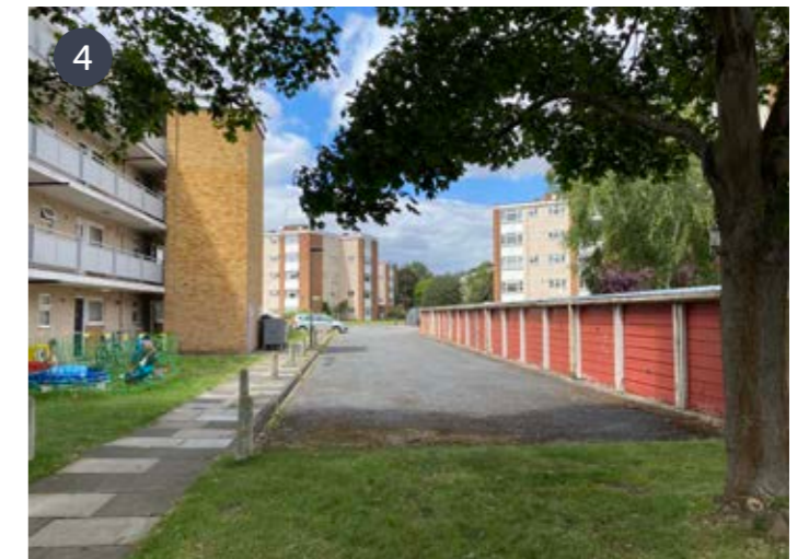
View to the rear of Grieg House from Ashburnham Road
