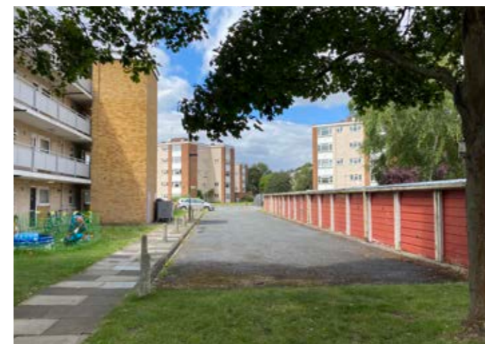
Garages and access close to Grieg House
