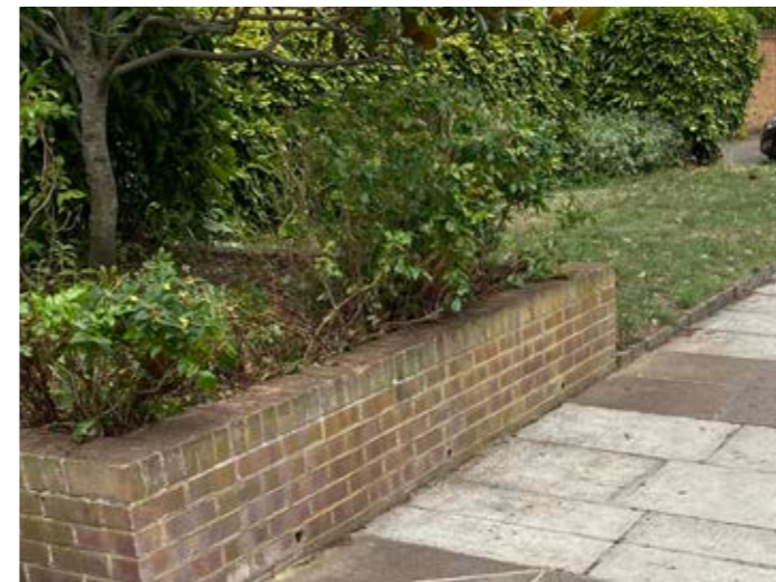
Raised planters to reinforce corners
