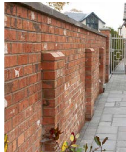
Typical brick wall - Western boundary & rear gardens
