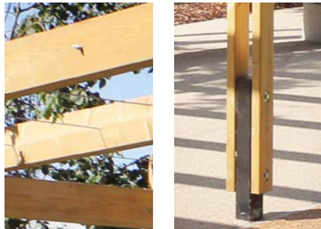
Slatted timber structure and metal shoe detailing
