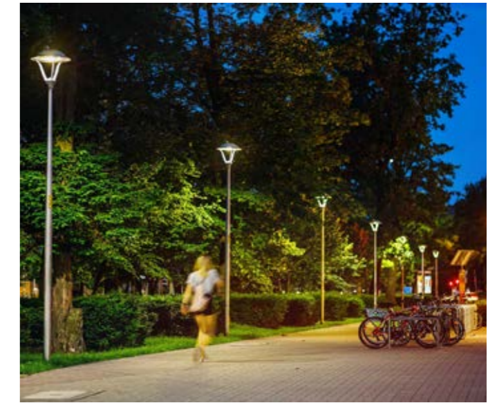
Column lighting to streets and courtyards.
