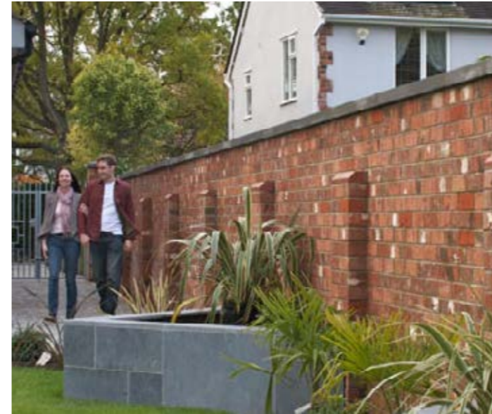
Traditional brick wall with piers and coping
