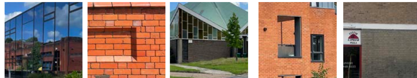
2 Large Span Window 4 Set Back Brick Detail 9 Differentiation of Material Recessed Terrace 1 Horizontal Banding
