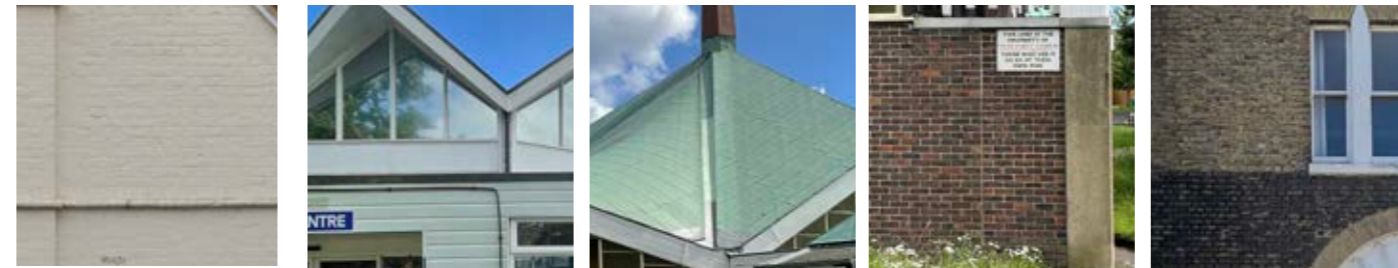
7 White Painted Brick 8 Green Painted Timber 9 Green Copper Roof 9 Dark Brick 9 Dark & Light Brick
