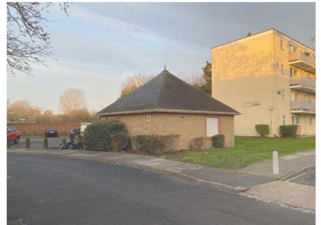
4. View of the existing Richmond MakerLabs facility
