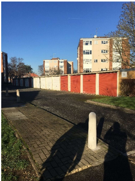
View of garages
