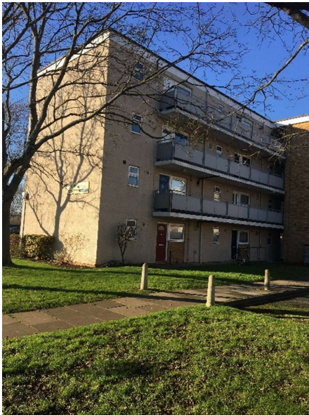
View of four storey block (Greig House).
