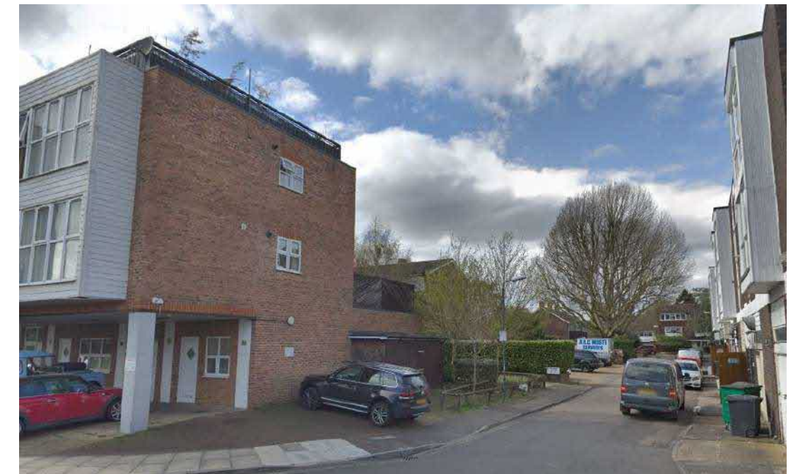
View from Ashburnham Road looking north west
