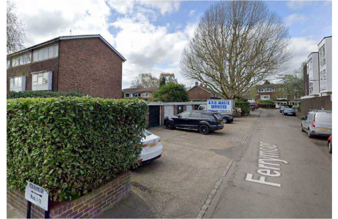
North view of the garages along Ferrymoor
