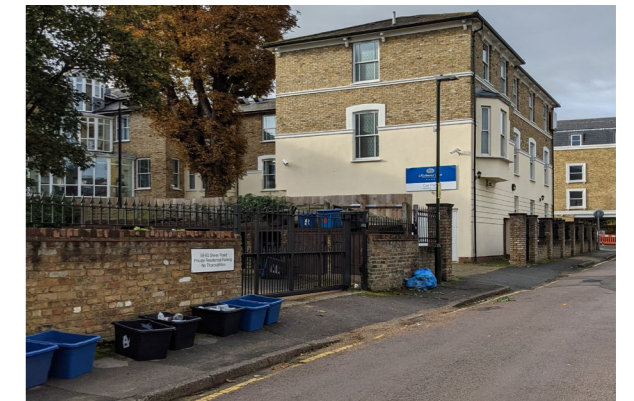
3. West facing view of the site from Sydney Road
