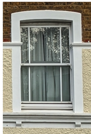
First Floor window on Sheen Rd
