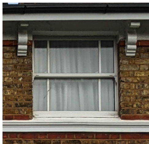
Second Floor window on Sheen Rd
