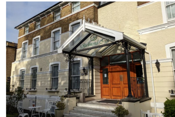
2. Entrance to the building from Sheen Road
