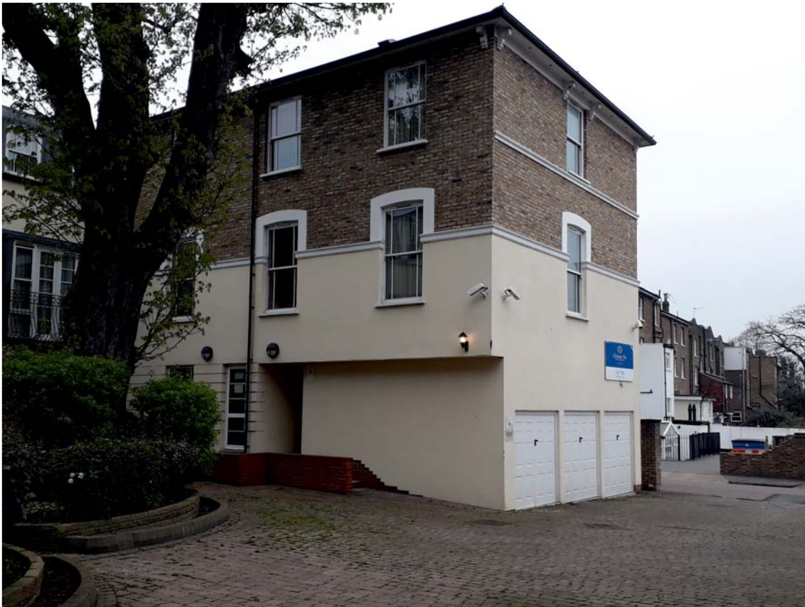
Fig 12 Carpark to the north of the hotel, looking north-west (MOLA photo, 30/03/2022)
