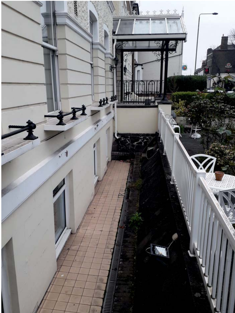
Fig 14 Richmond Inn Hotel, front of the building showing lightwell and windows into lower ground floor, looking east (MOLA photo, 30/03/2022)
