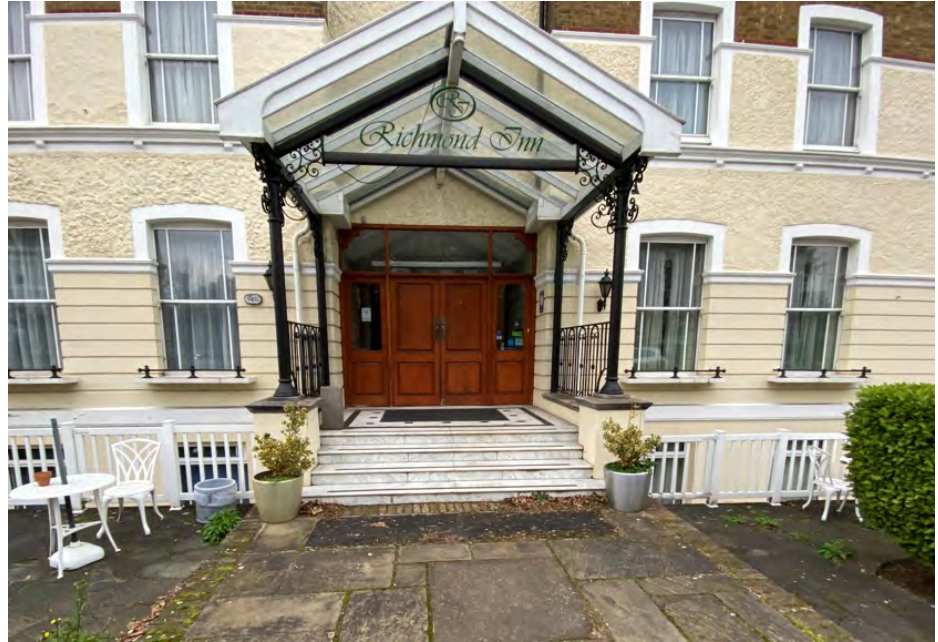
Figure 12: Sheen Road entrance
