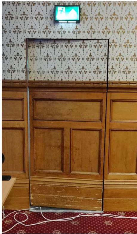
Figure 8 - The second non-original fire exit door. We wish to recreate a wider version of this door of a similar design.
