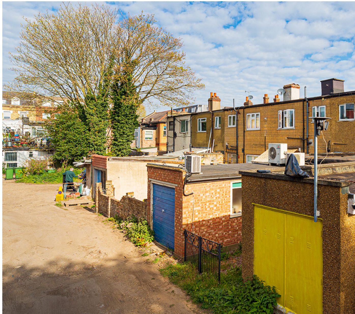
FIGURE 12 - EXISTING VIEW OF REAR (NO. 3-4 IN STONE CLADDING)
