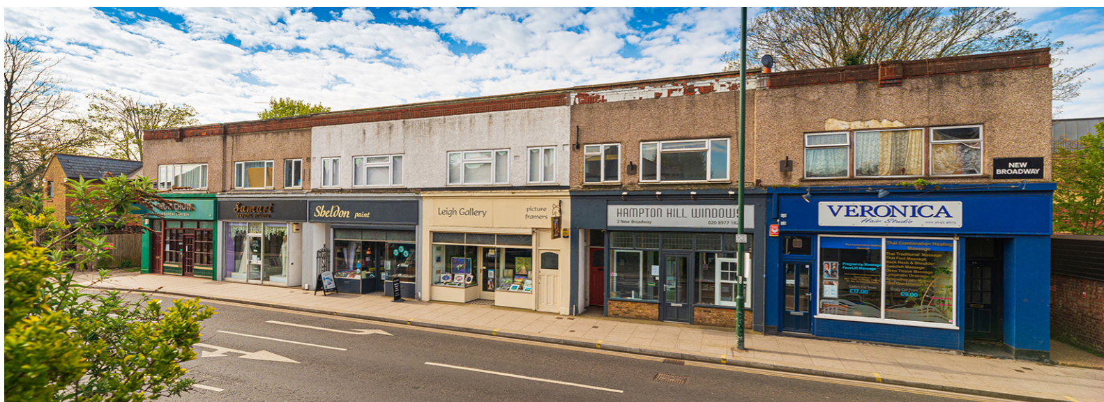
FIGURE 04 - EXISTING 1-6 NEW BROADWAY (NO. 3&4 IN MIDDLE)
