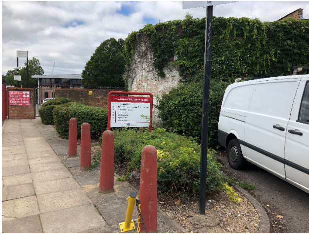
Photograph 3.5 Ivy clad wall on western site boundary
