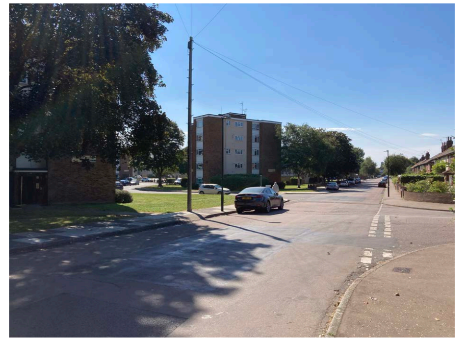
Figure 6.7: Ham Close as seen from Woodville Road.
