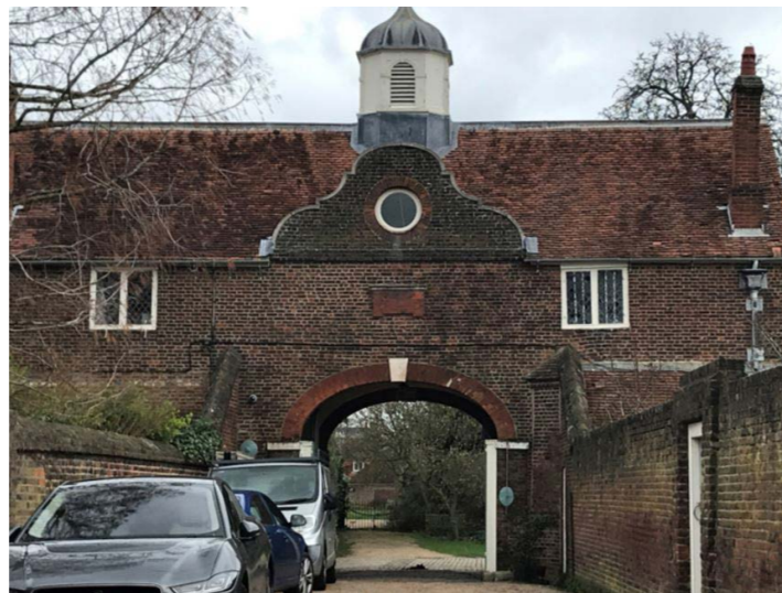
Figure 6.34: Ham House Stables. Source: Historic England website.
