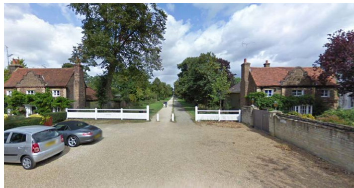
Figure 6.44: Avenue Cottages. Source: Google 2022.
