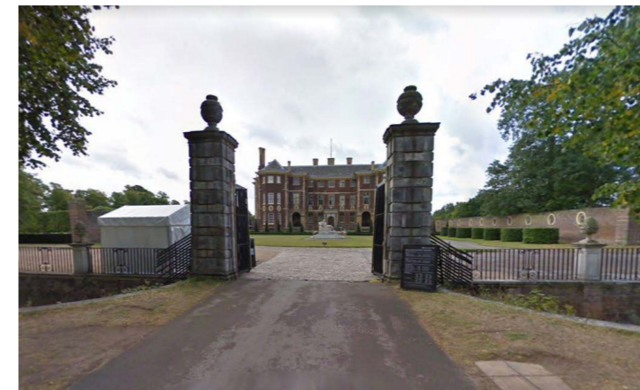
Figure 6.31: Entrance, gates and railings of Forecourt to Ham House. Source: Historic England website.
