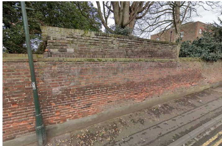
Figure 6.41: Boundary Wall to Beaufort House. Source: Google 2022.
