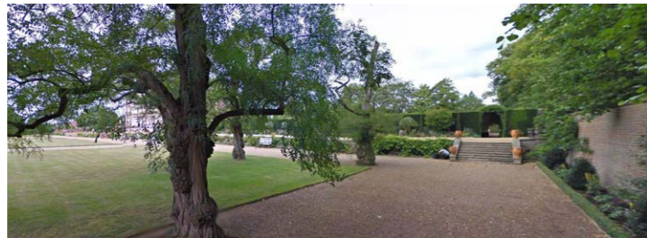
Figure 6.33: Garden Walls and Gate-piers to south of House. Source: Google 2022.
