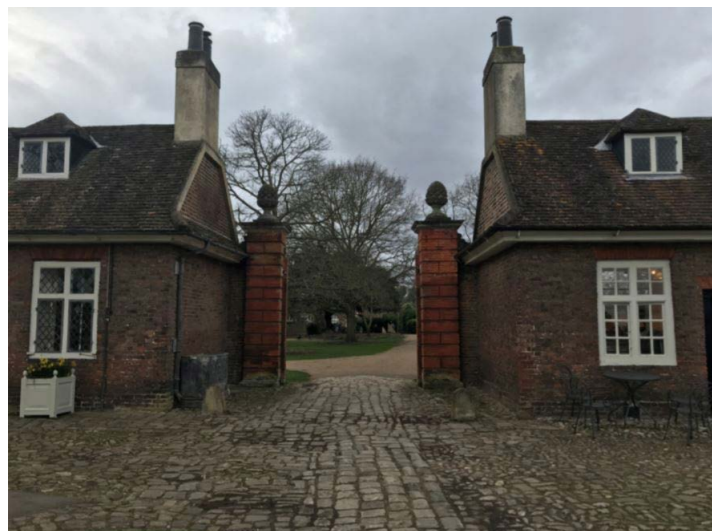
Figure 6.36: Service Yard Entrance to West of House. Source: Historic England website.
