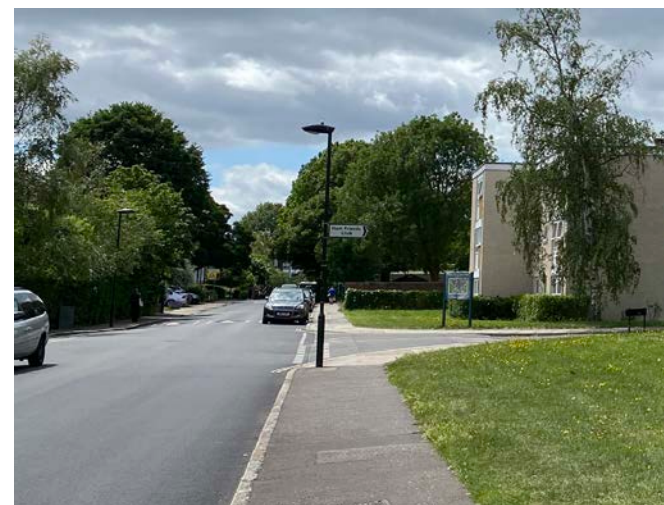
Existing lighting columns on Ashburnham Road
