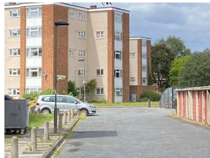
Existing lighting columns within Ham Close parking areas
