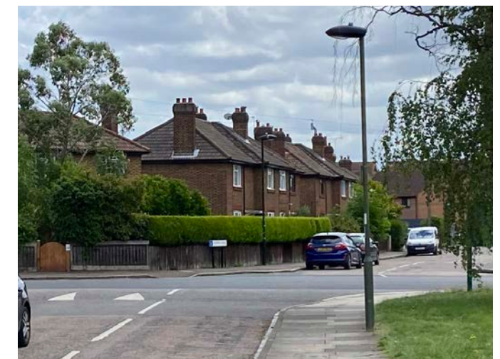
Existing lighting columns on Ham Close
