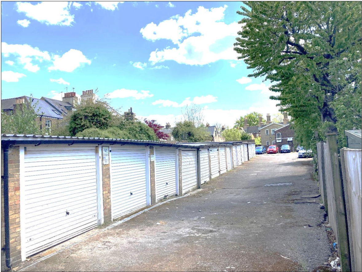
Fig. 1 St Mary's Grove Garages looking south
