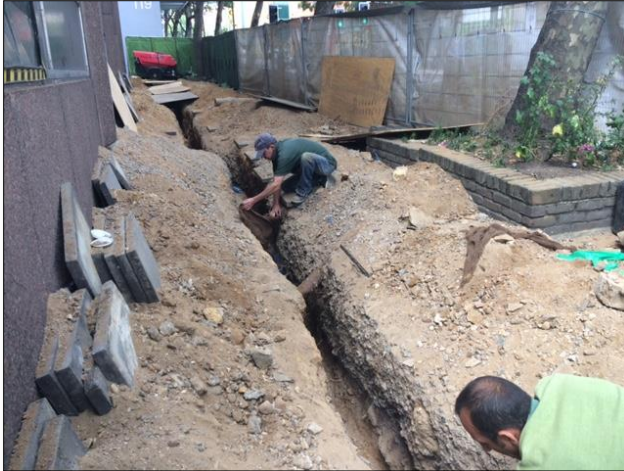
Fig. 2 Use compressed air to remove soil from roots
