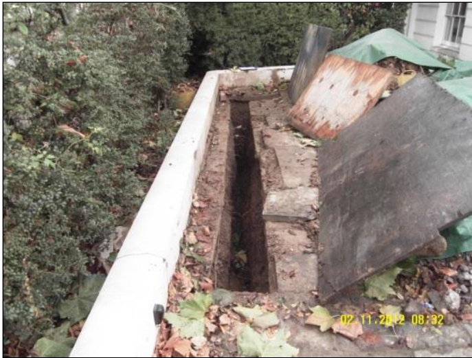
Fig. 3 Lift pavings and use boards to cover pits and trenches for safety
