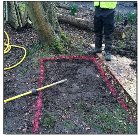
Fig. 1 Protect the site (left) and mark out the area for excavation and lay ground protection
