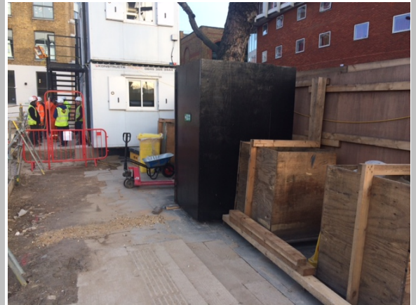
Robust hoarding and temporary concrete ground protection
