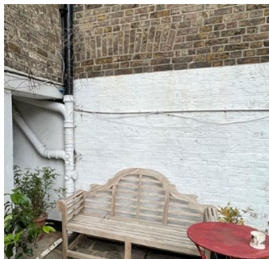
Ground Floor Window – Blocked Up – showing original soldier course brick lintel.
