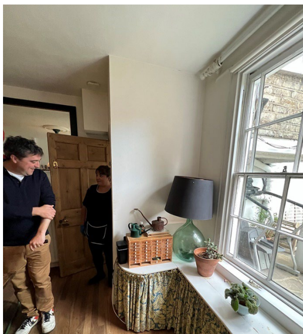
Modern partition and soil pipe boxing (top left) to be removed – returning room to original configuration.
