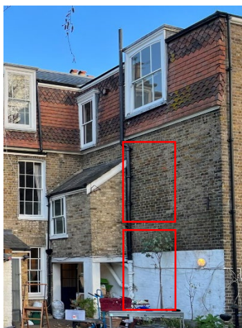
Georgian Rear elevation showing location of two blocked up windows.
