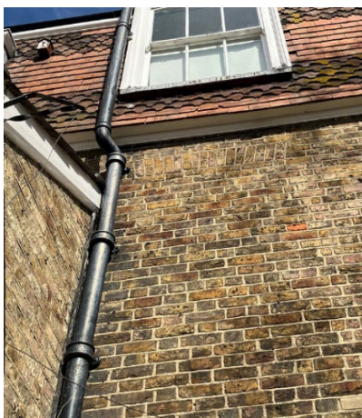
First Floor Window – Blocked Up – showing original soldier course brick lintel.
