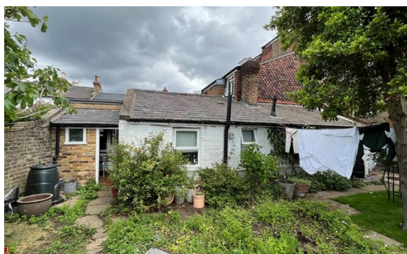
Outbuilding showing set back utility/wc extension to left.
